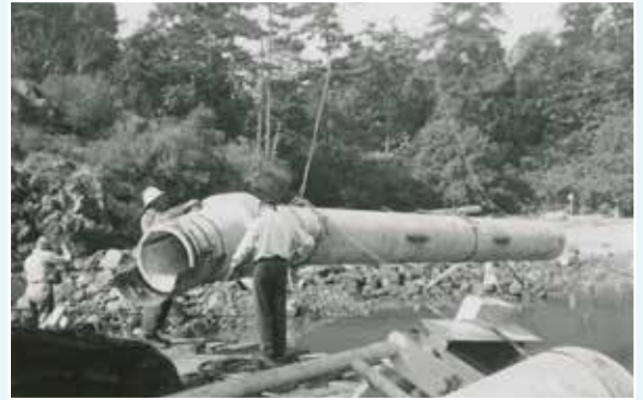
1980-015-258c Construction of Arbutus Outfall 1955
